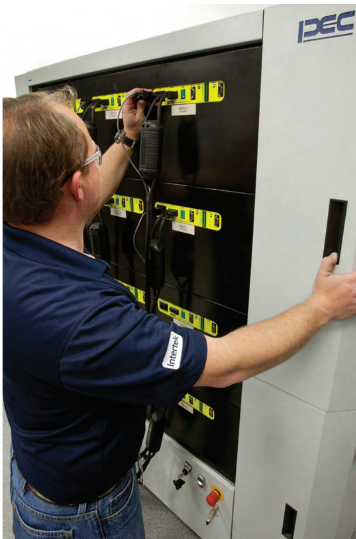
Engineer Kirk Palmer attaches a voltage sensor connector to the PEC 8050 in order to monitor voltage levels during the testing of a battery
